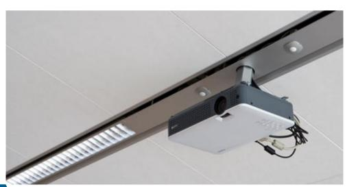
To add to the feeling of calm and simplicity, the architect firm C.F. Møller developed a lighting strip for the ceilings which contains both lighting and ventilation in the same band, contributing to the orderly feeling of the ceilings.
