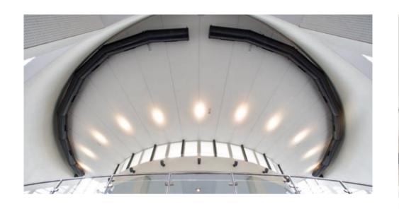
A substantial proportion of the total space comprises a large indoor swimming pool, sauna, fitness facility and spa in the wellness centre. The relatively high humidity level in these areas made Rockfon Sonar's high resistance to moisture a key element while maintaining the high design level.
