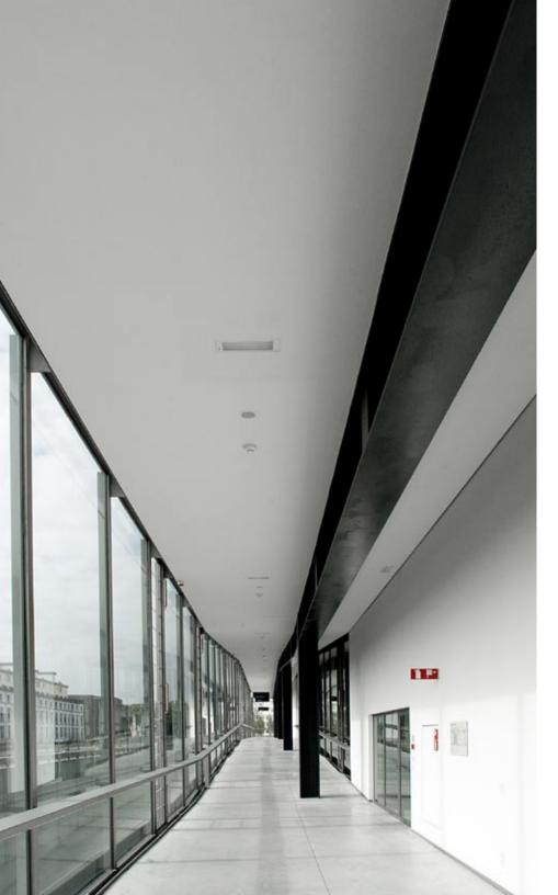
The Mono Acoustic system comprises a suspended system to which Rockfon ceiling panels are secured using screw plates. The joints are concealed with a filler and then sanded. Once the ceiling is completely smooth, it is finished with a spray plaster which creates the seamless appearance.
