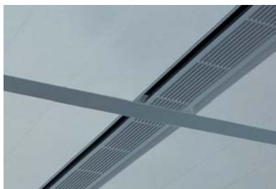
Chilled beam unit integrated into OWAcoustic® bandraaster ceiling.
